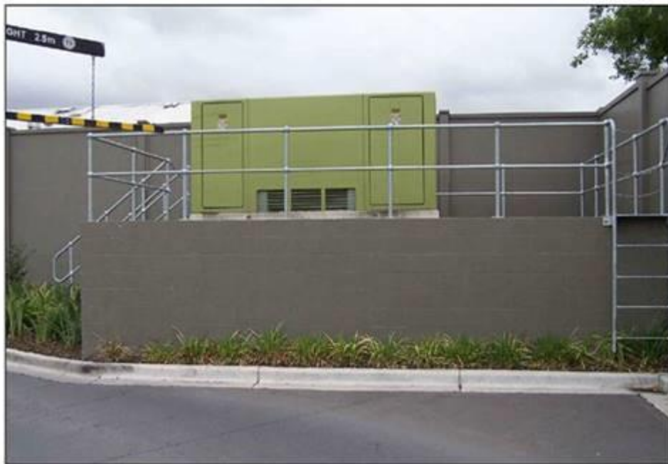
Figure 51 - Example substation raised above 1:100 flood level
